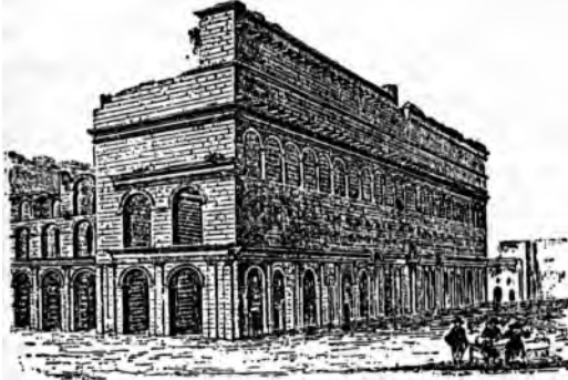
FIGURE 134. EXTERIOR OF THEATER AT ORANGE
